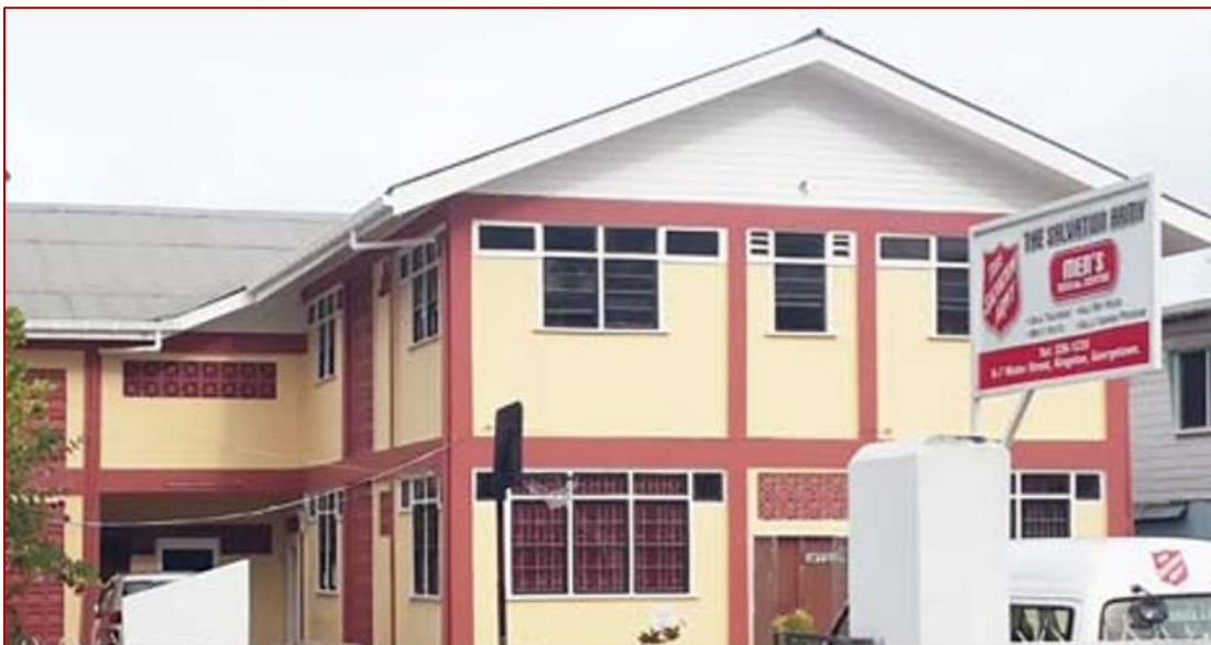
The Salvation Army- Men's Social Service, Located: 6 Water St. Kingston, Guyana, Phone: 592-226-1235
